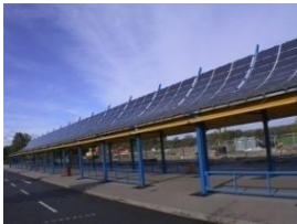
Europapark Rust, 250 kW
